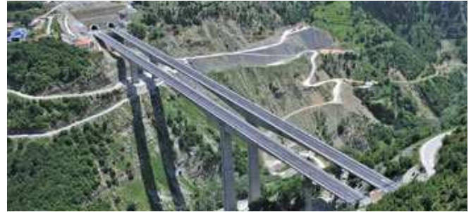
The Metsovitikos Bridge connects two tunnels along the Egnatia Motorway.
