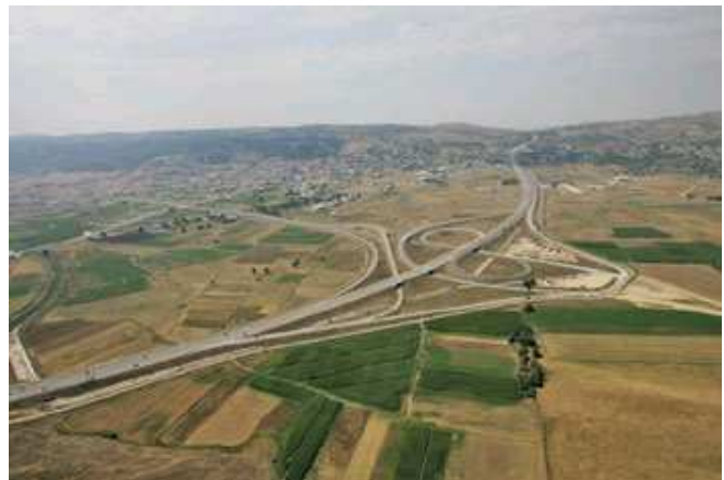
This new interchange near Thessaloniki is one of nearly 60 new interchanges along the 416-mile (670-km.) Egnatia Motorway in Greece.
