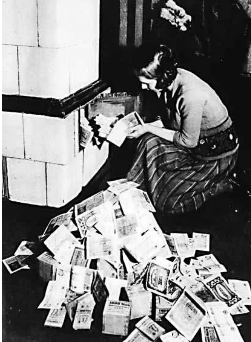
Burning marks as fuel to keep warm. Germany, 1913.
